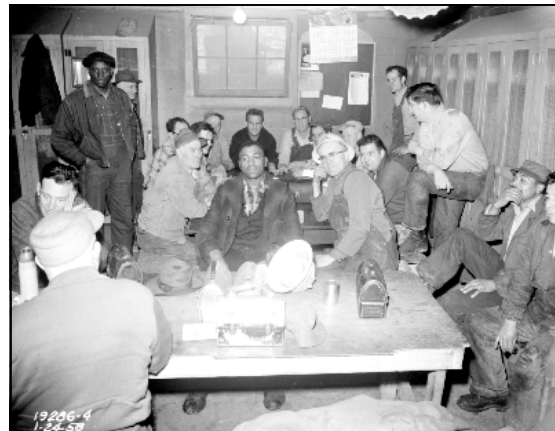
Asphalt workers in the crowded Charles Street Shop break room, January 1958
