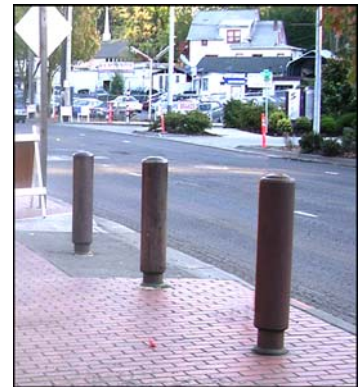
Cast iron bollards in Columbia City incorporating 19 th Century theme
