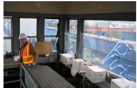
Interior view of an unused Fremont Bridge tower.
