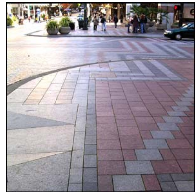
Granite Unit pavers at Westlake Center
