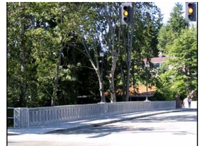
SDOT's historic reproduction on Princeton Bridge
