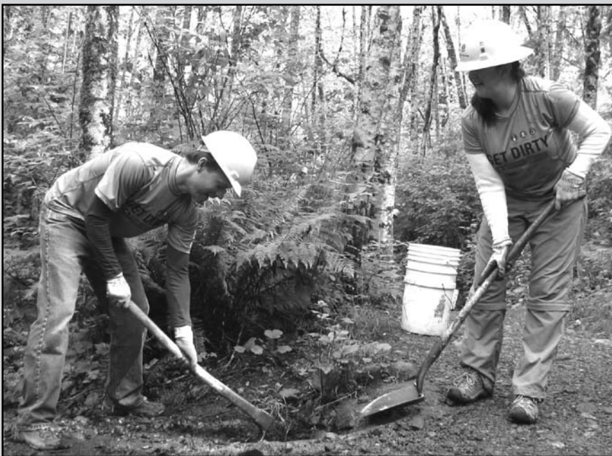
Two Greenway volunteers from REI remove sediment from a culvert to keep water off the Twin Falls trail. More than a dozen volunteers from REI worked on this popular trail in Olallie State Park on National Trails Day.
