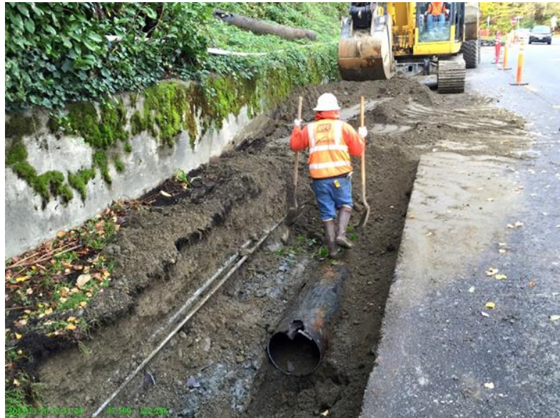
Figure 4-4. Combined Sewer Replacement in Leschi
