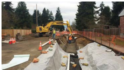
Inline storage (in construction)
