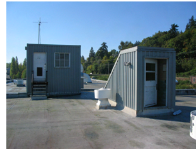
Existing Rooftop Equipment Structures
