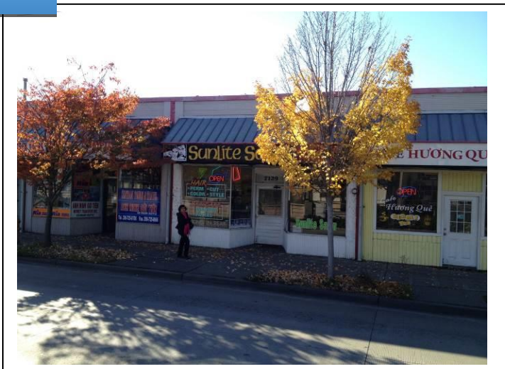
7129 – Sunlite Salon Storefront Observations: retain use, remodel, facelift
