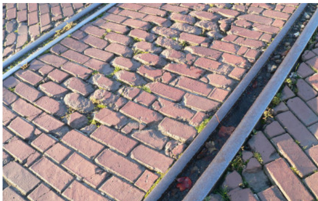
Unused “orphan” tracks are located along Utah Avenue S and in other parts of SODO.
