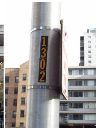
Each overhead light has a light pole number.
