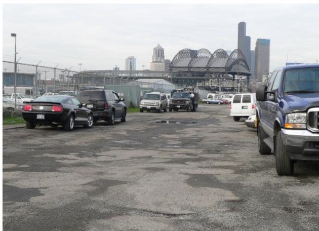
Poor pavement conditions on 3rd Avenue S
