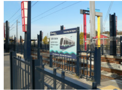
The SODO LINK light rail station.
