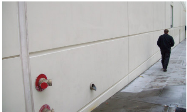
Blank walls can contribute to poor CPTED design.
