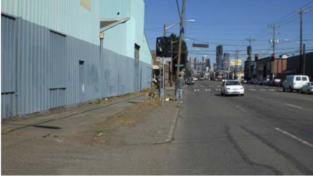
Example of poor condition of sidewalk and driveways, including driveways no longer in use.
