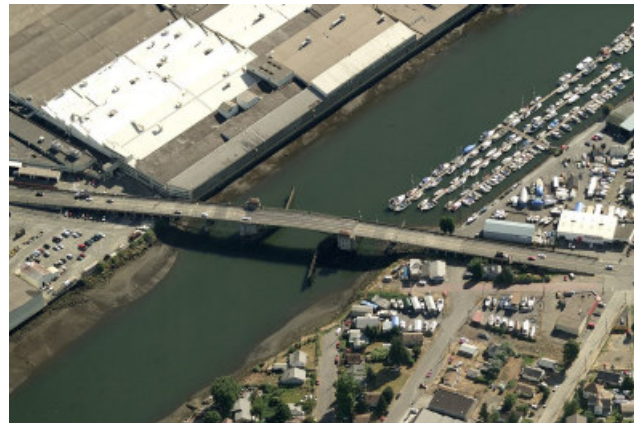
South Park Bridge
