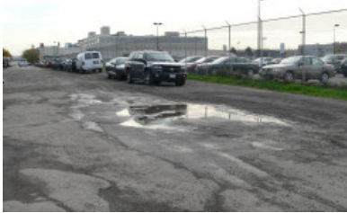
Pavement conditions on 3rd Avenue S.
