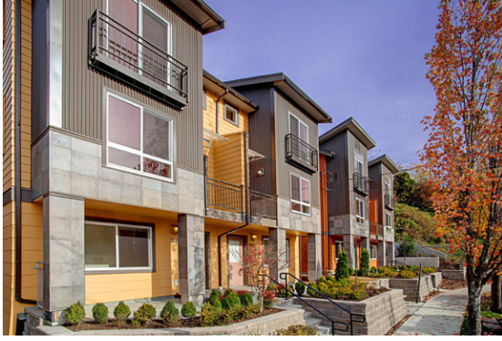
Nova Townhomes, community land trust affordable housing near the International District.
