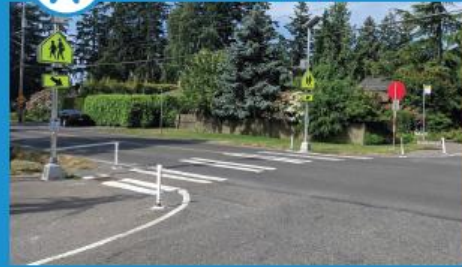
Installing crossing improvements
