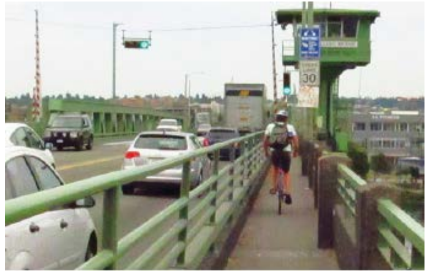
Existing railing near bascule portion
