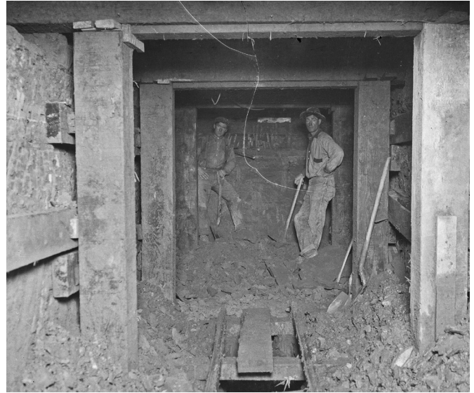
Excavating by hand for a new sewer line in 1912.
