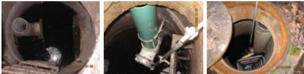
Detention System (Flow Control Structure)
