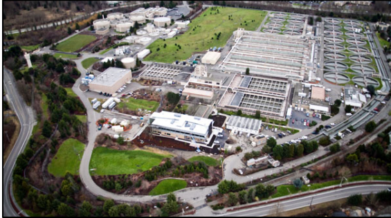
South Treatment Plant
