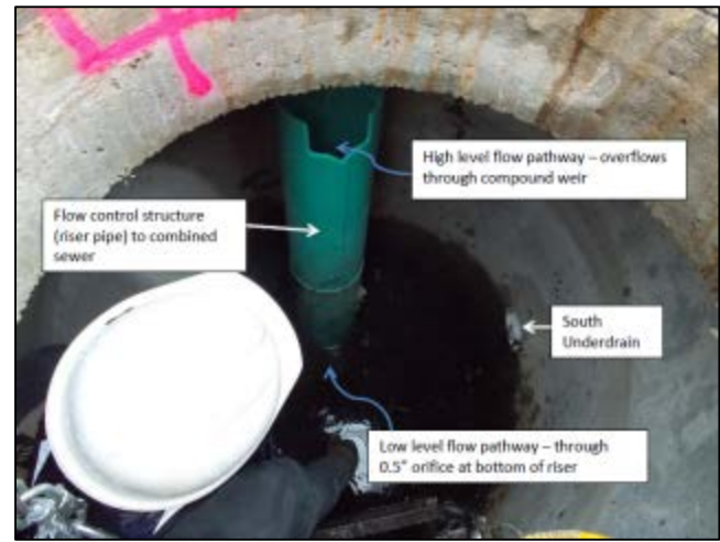
Figure 16b. MH 4 Flow Control Structure Riser Pipe
