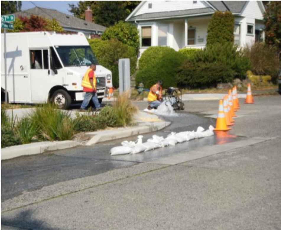
Figure 18. Controlled Flow Testing on 28th Avenue NW at NW 67th Street
