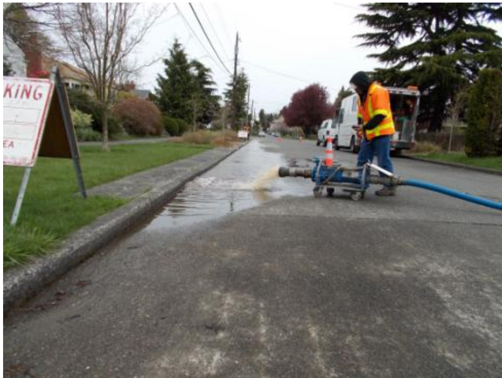
Figure 17. Controlled Flow Testing at the 30th Avenue Rain garden (looking north)
