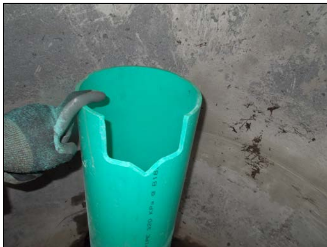
Figure B-2 – Thel-Mar Overflow Weir in MH 4 at the 28th Avenue Raingarden.
