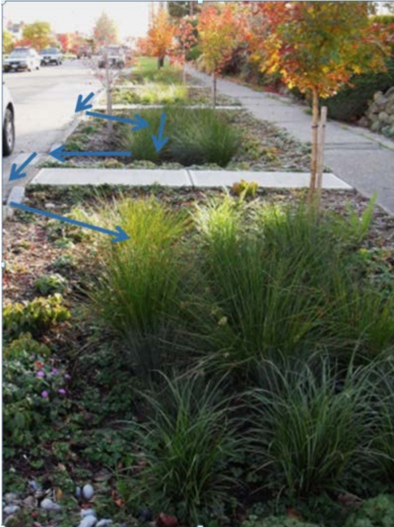
Figure 5. Typical Flow Pathway through the 30th Avenue Raingarden
