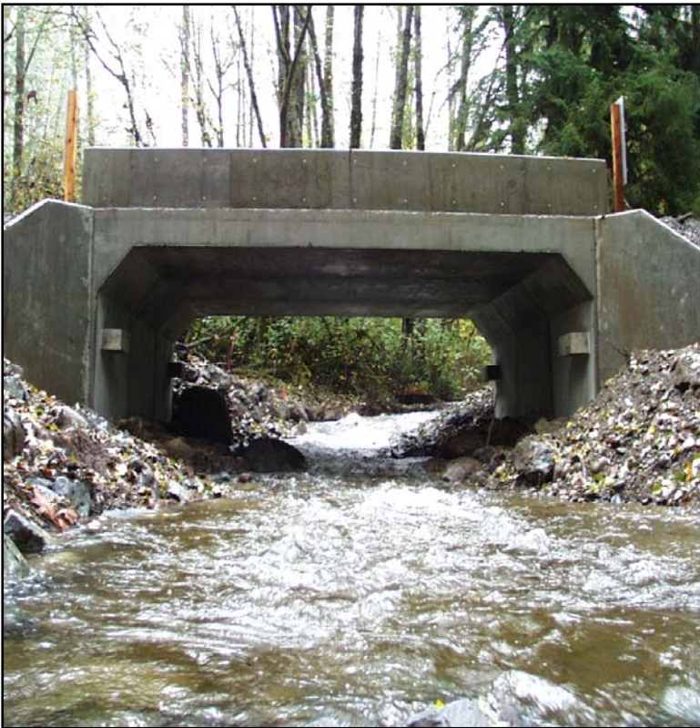
Webster Creek 10 Road following bridge installation in fall 2001.
