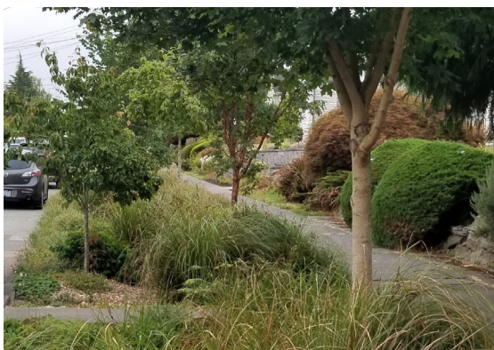
An example of a completed natural drainage system on a residential street.
