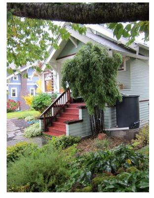
Figure 4-2. Raingarden (left) and Cistern (right)
