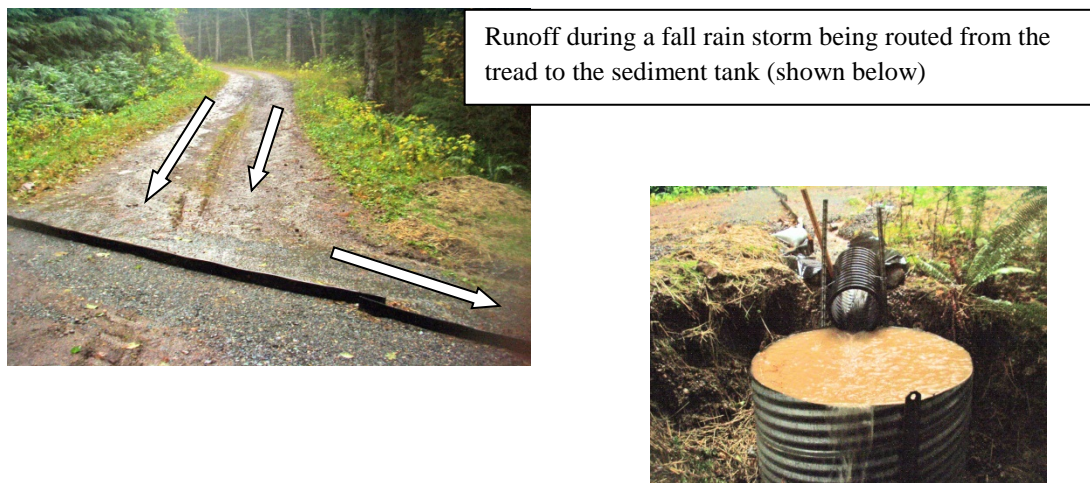
Figure 5. Sediment tank and tread diverter setup.
