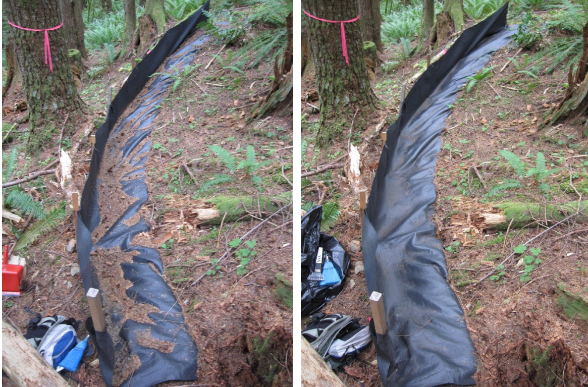
Figure 8. Typical silt fence site before and after collecting sediment for measurement.
