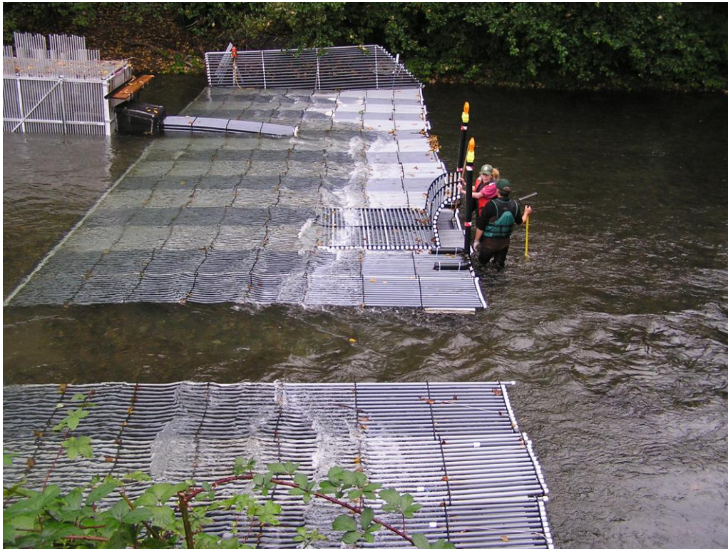
Figure 1, Floating Resistance-Board Weir and Trap with 2 Panels Pulled to Allow Unimpeded Upstream Fish Passage.
