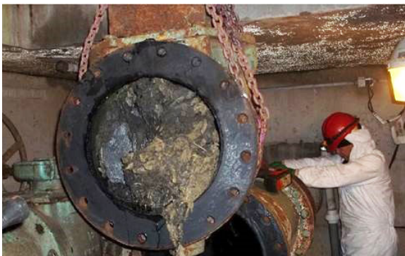
Wipes cause major blockages in Seattle's sewer system, like this pile of wipes clogging a pump station in SE Seattle.
