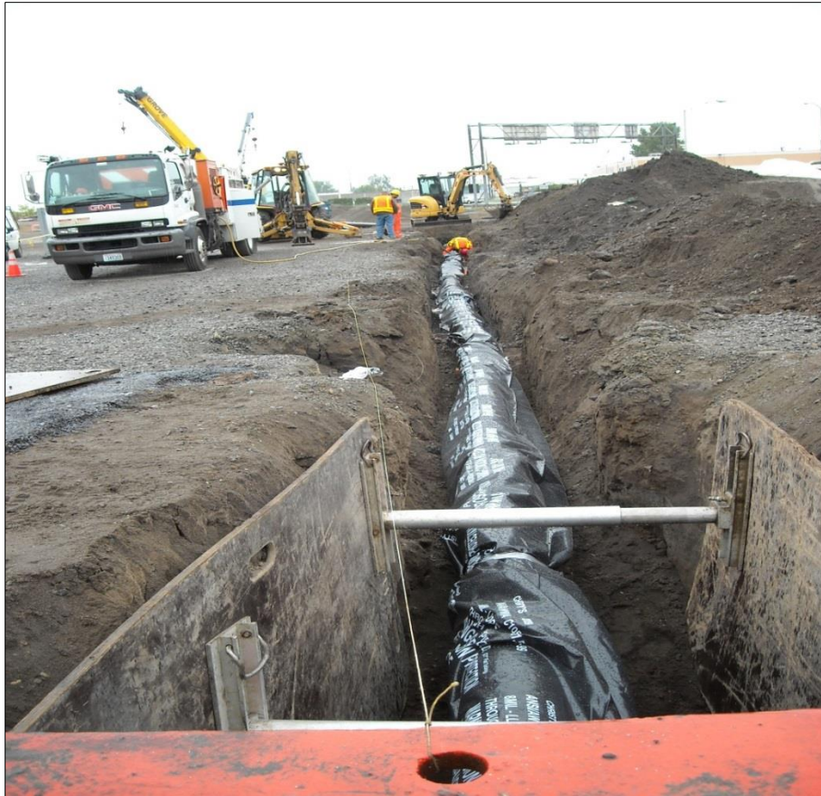
South Transfer Station 8" water main
