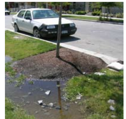
grading adjustments are needed where extended ponding occurs
