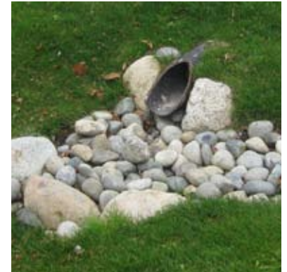
cobbles placed in erosion-prone area near outlet pipe
