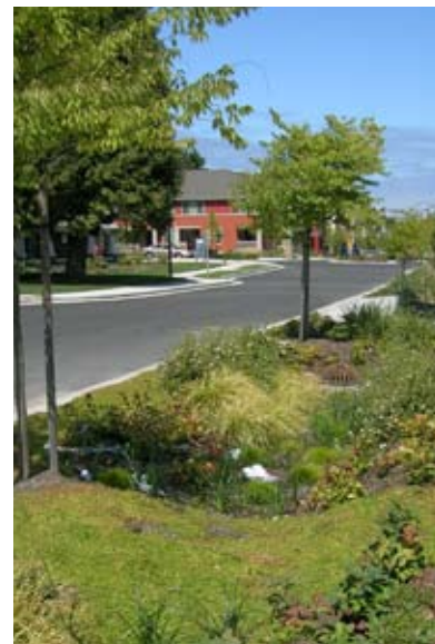
debris in swale
