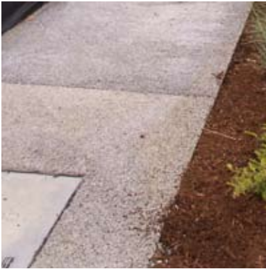
soil and mulch deposited on a porous cement concrete walk
