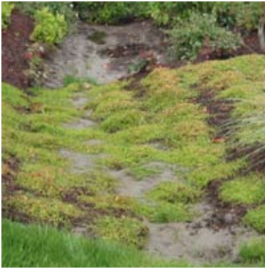
erosion and sediment build-up in swale
