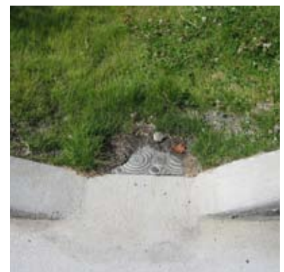
curb cut inlet art requires sediment removal
