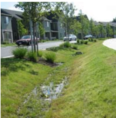
ponding at swale bottom
