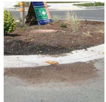
washout from planting area onto street
