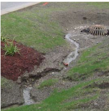
channeling and erosion in grass swale
