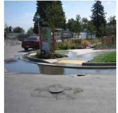
irrigation overspray and day time watering necessitate irrigation adjustments.
