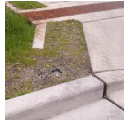
worn reinforced grass edge
