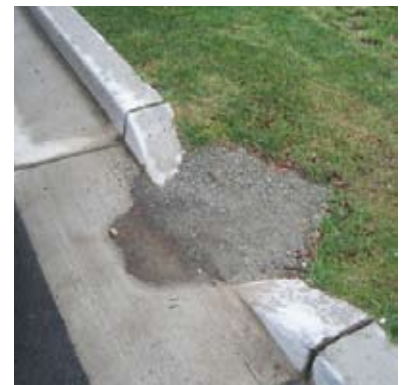
examples of sediment build-up in drain curb cut openings
