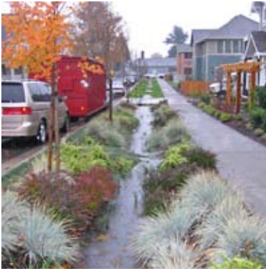
overflow channel and pedestrian berm
