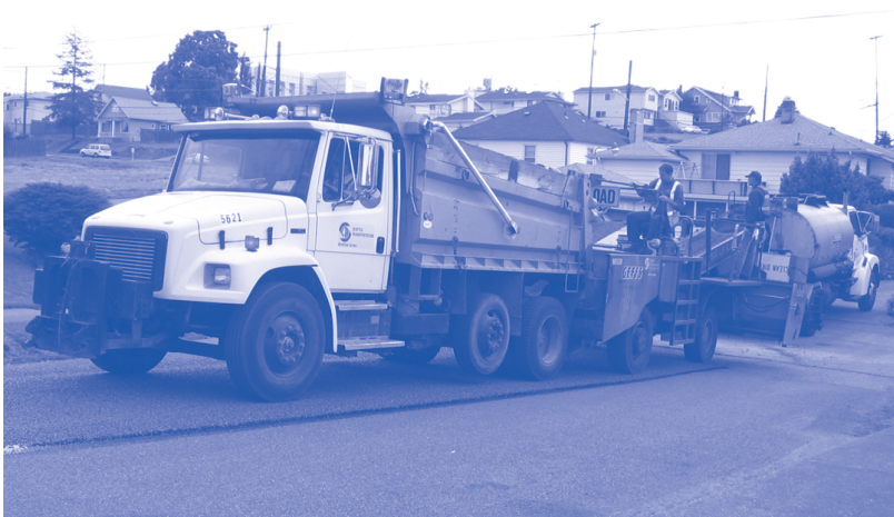
A street being chip-sealed. SDOT uses chip-sealing, a low cost and highly effective surface treatment, to preserve and maintain many of Seattle's non-arterial streets.
