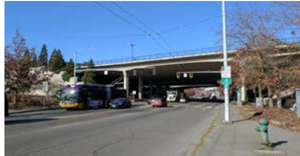
Rainier Ave is a constrained right-of-way that primarily serves freight, buses, and other vehicles and, in this area, connects drivers to I-90.
