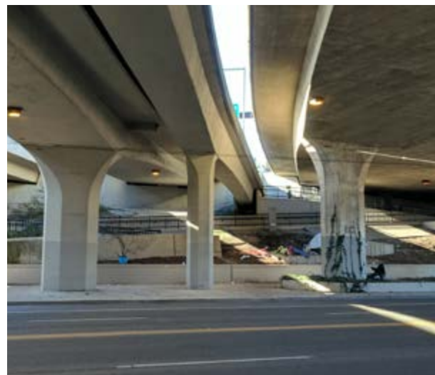
The future light rail station's west entries will be located on Rainier Ave S at this I-90 overpass.
