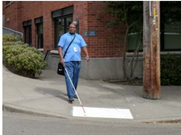
Tactile paving alerts a Lighthouse for the Blind employee that he is leaving the sidewalk and entering the street.
