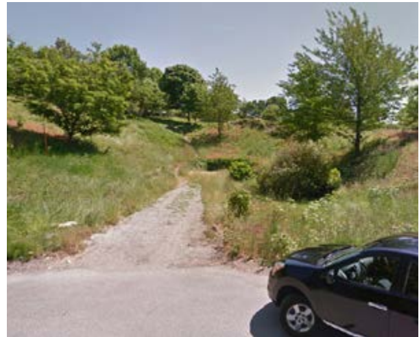
Existing footpath between Hiawatha Pl and MTS-Dearborn Connector Trail
