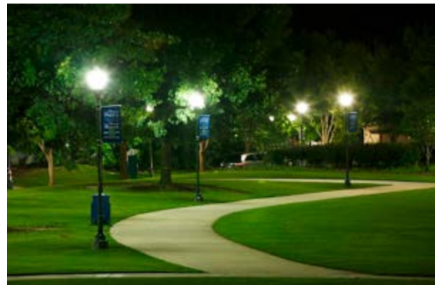
Closely spaced, low level, pedestrian lighting would improve trail safety and sense of security.
