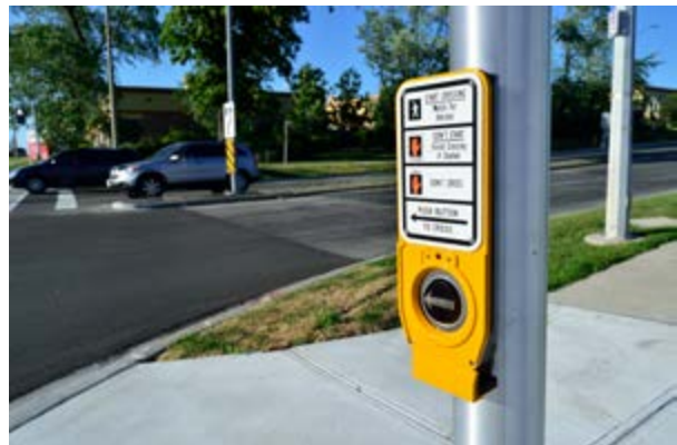
Tactile and audible accessible pedestrian signals (APSs) help people align to the intersection and know when it is safe to cross.
