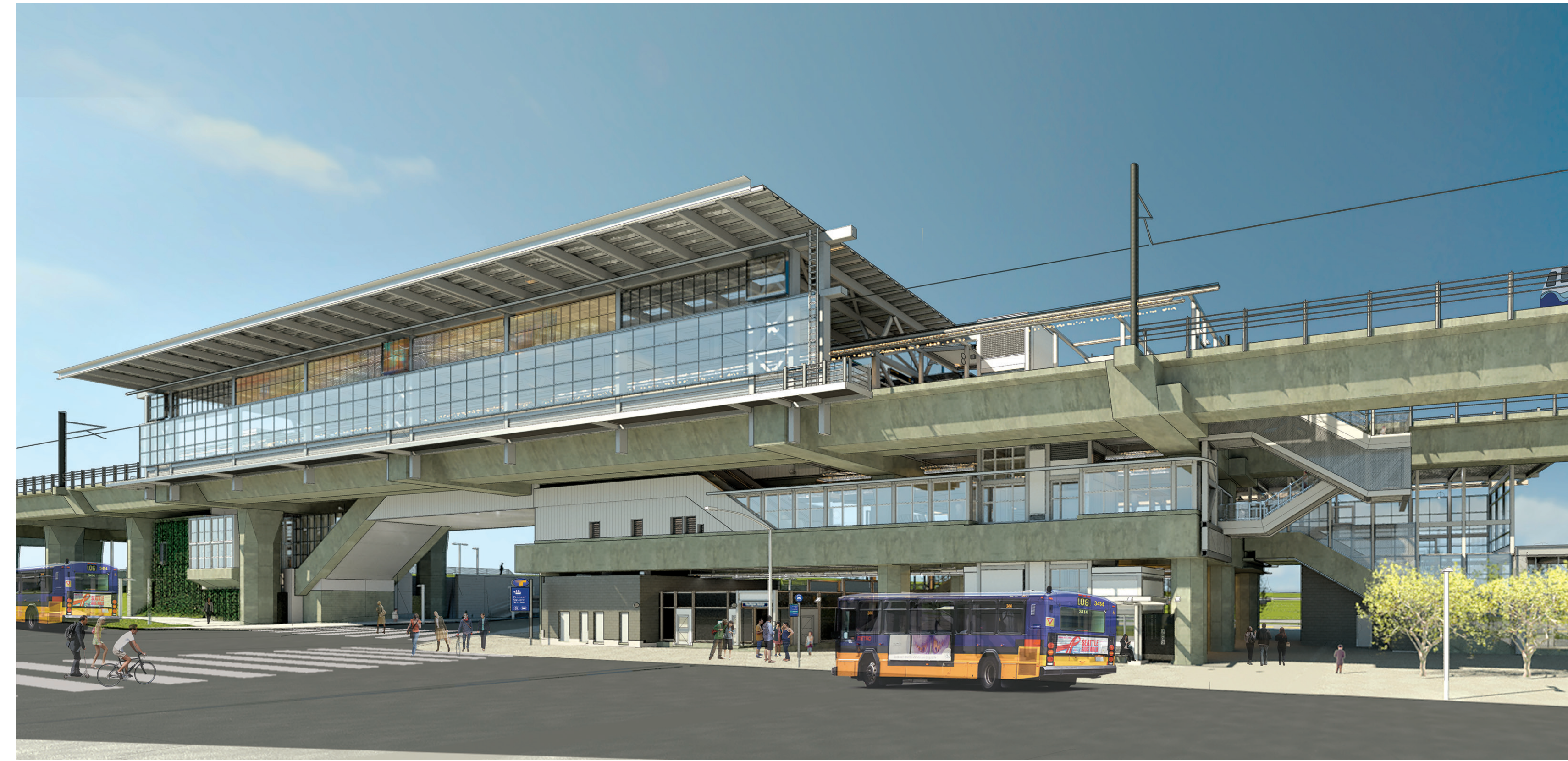
Northgate Transit Center Station
