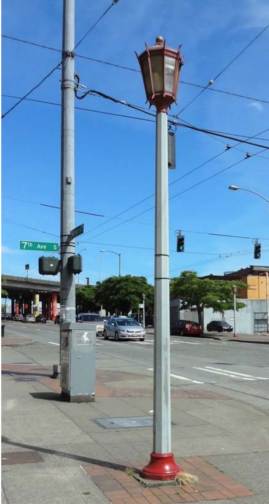
Figure 2 Pedestrian Light Pole
