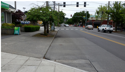
Looking south from the RapidRide stop on the east side of California Avenue SW north of Fautleroy Way SW
