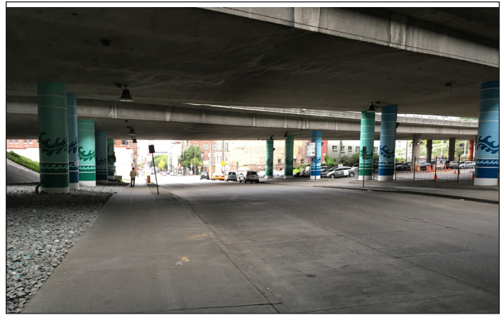
Looking west underneath I-5 underpass
