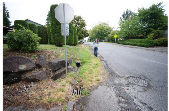
Existing conditions at NE 135th St and 35th Ave NE - Northeast Corner
