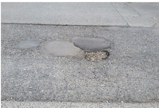
Looking eastward at a pothole in the asphalt section of the 8th Ave S near S Chicago St
