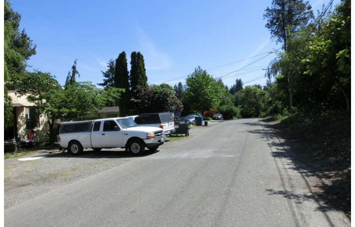
There are no existing sidewalks on NE 85th Street.
