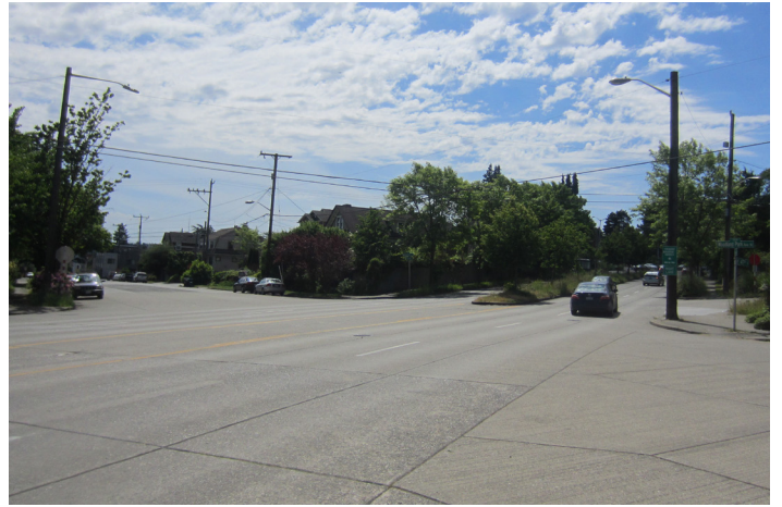
Existing conditions looking south to Woodland Park Ave N from Green Lake Way N
