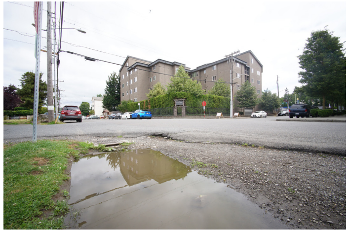
Existing gravel and paved shoulders lack drainage infrastructure.
