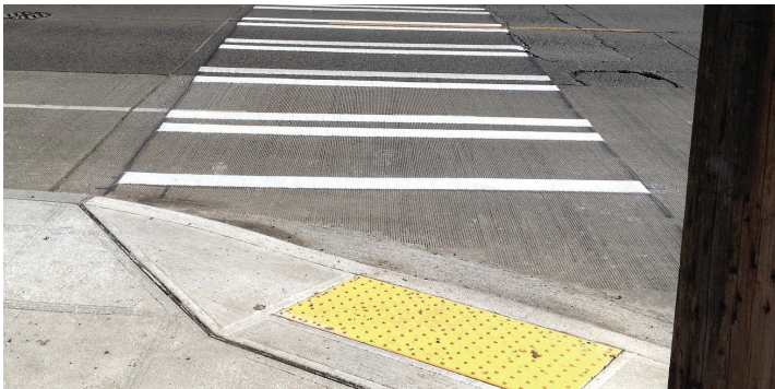
New or upgraded curb ramps at some intersections along N 80th St.
