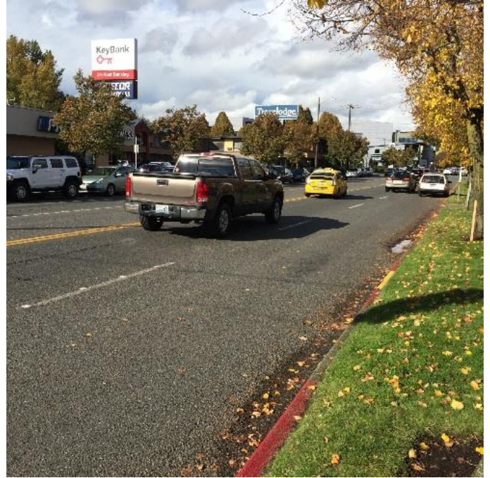
25th Ave NE needs to be resurfaced and restriped
