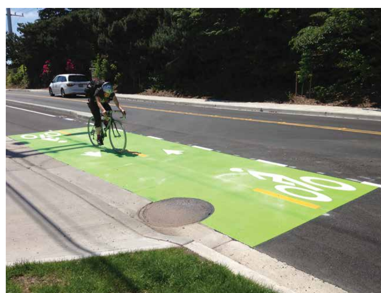
Bike Lane Visibility at Driveways
