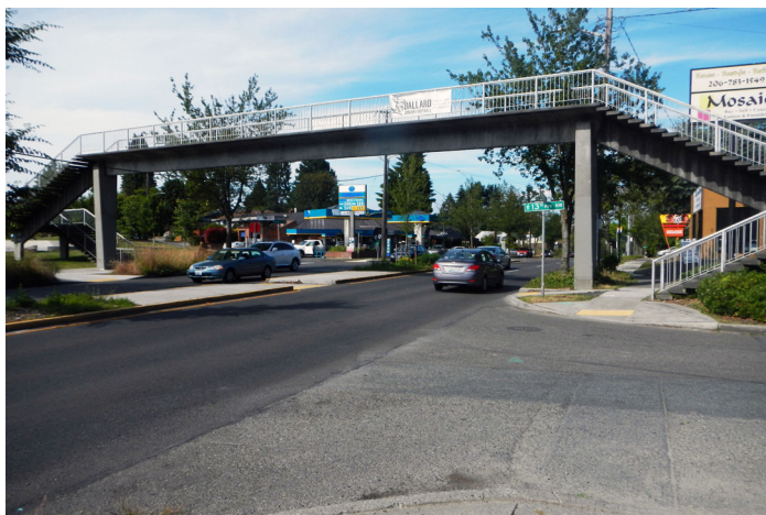
Existing conditions at Holman Road NW and 13th Ave NW intersection
