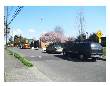
Speed humps are about three inches high and 12 feet long. They support a 20 mph speed limit and discourage cut through traffic.
