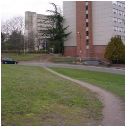
The lack of adequate pedestrian facilities (such as sidewalks) on the north end of the University Bridge is highlighted by the worn-down path that crosses the NE 40th St loop ramp. Inadequate lighting also contributes to a lack of pedestrian comfort and safety.
