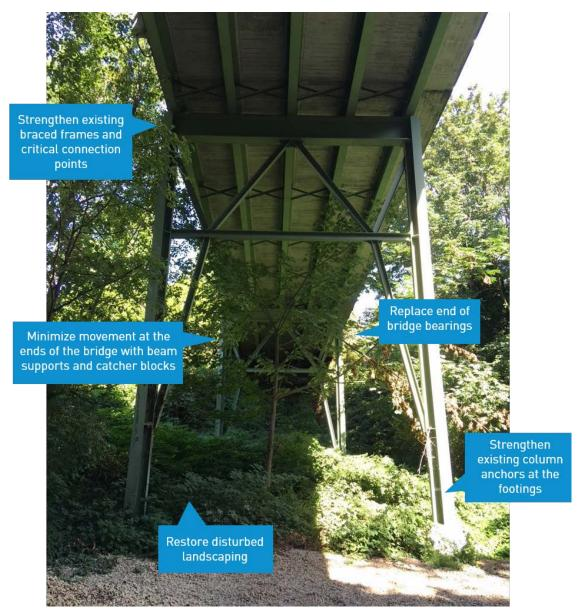
Photo of the underside of W Howe St Bridge with descriptions of planned seismic retrofits
