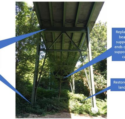
Replace end of bridge bearings; Stabilize support beams at the ends of the bridge with support beam caps and catcher blocks
