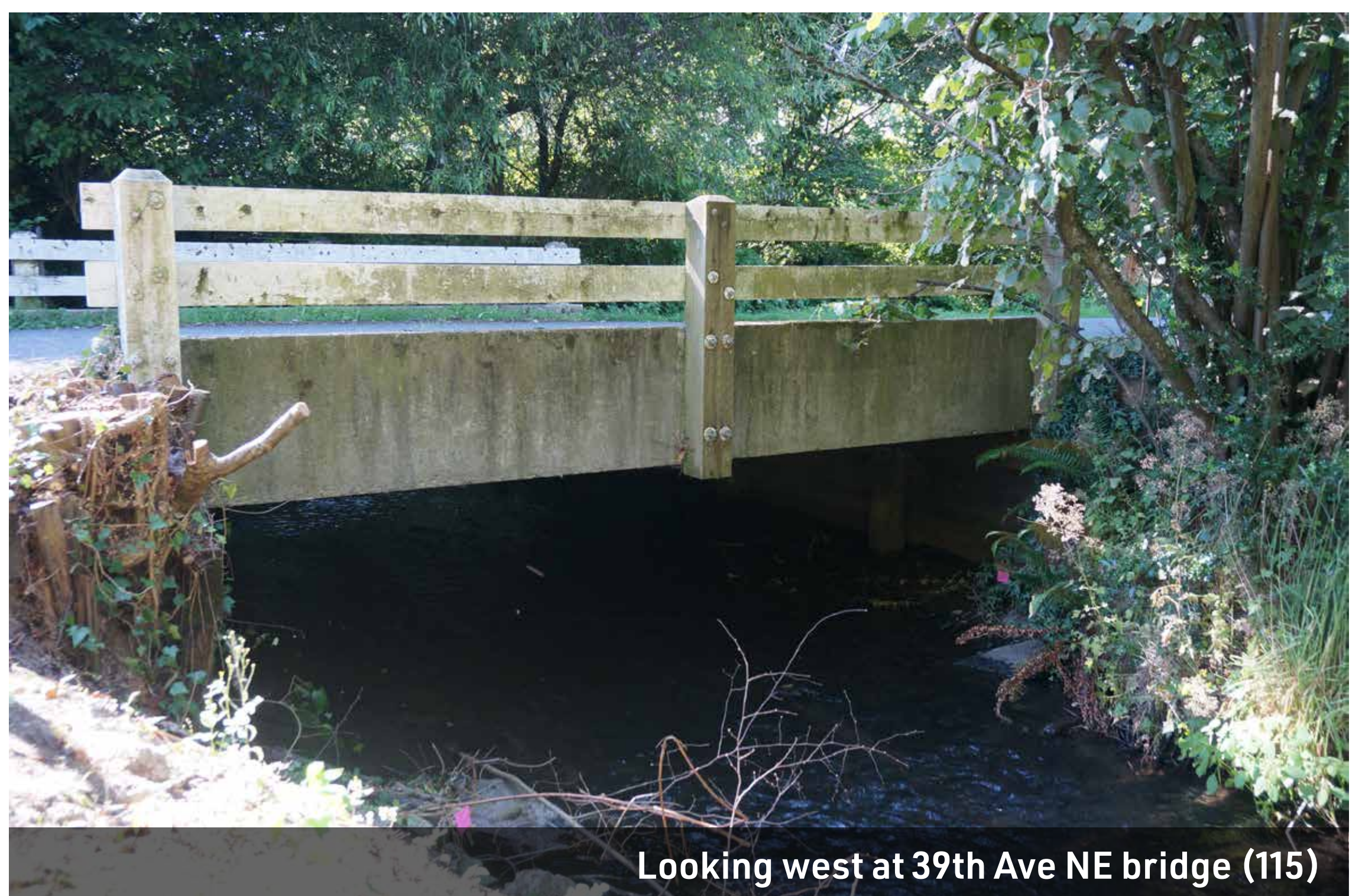
Street view of 39th Ave NE bridge (115)
