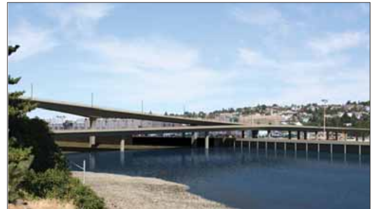
A photo simulation of how the new Magnolia Bridge will look [Haunched Cast-in-Place Concrete Box Girder (Main Structure); Precast Concrete Box Girder (Ramp Structure)]
