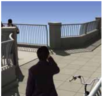
Steel tube railing and a concrete half-wall will border the bridge's sidewalk
