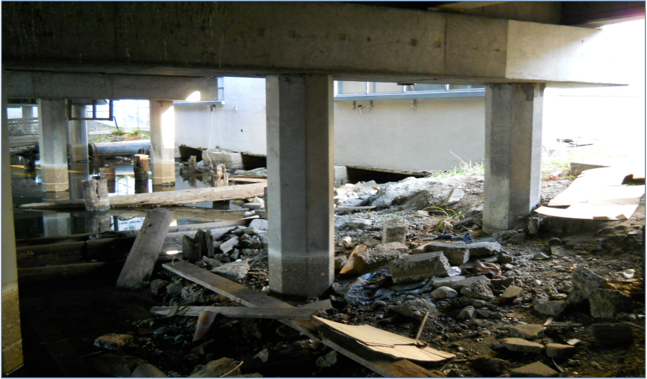
Photo 5. View under existing East Bridge, looking northerly. Note concrete piles and large amount of concrete rubble, wood waste, and garbage currently under bridge. This material would be removed as part of the project.
