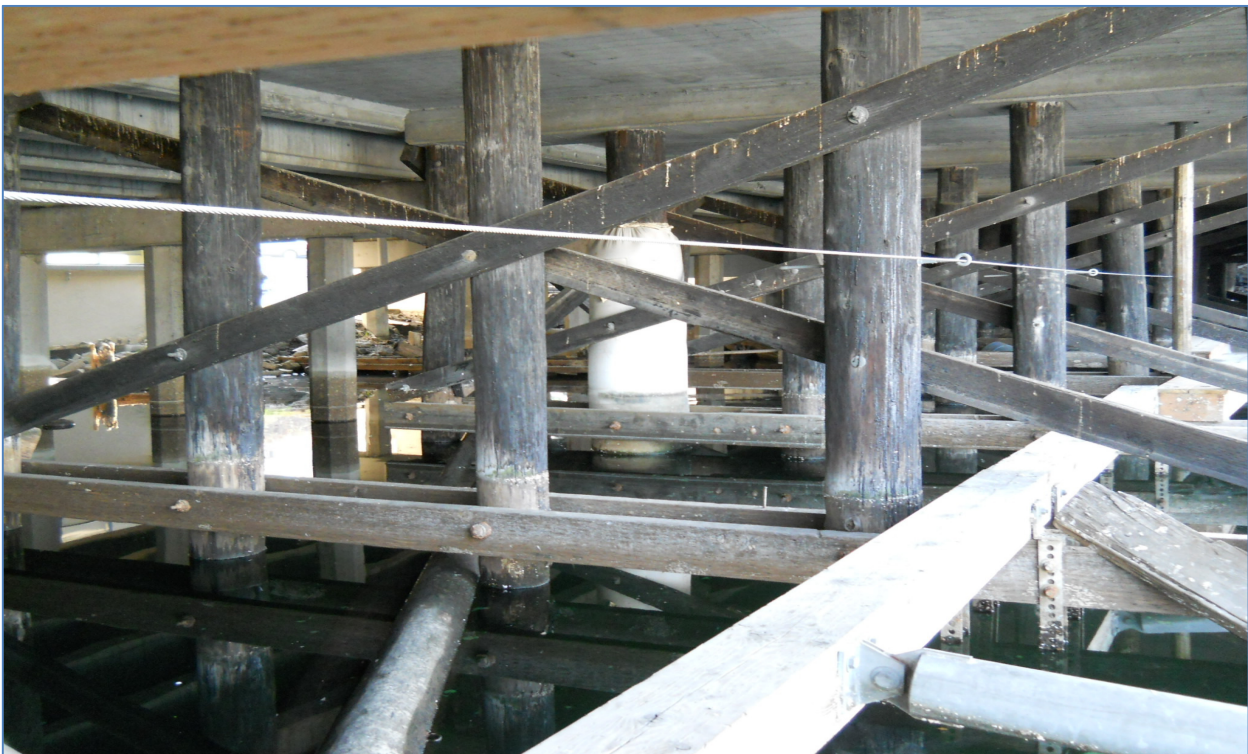
Photo 4. View under existing West Bridge, looking southerly. Note creosote treated piles and wooden bracing. Attachment system for floating walkway is shown on the right side of photo.
