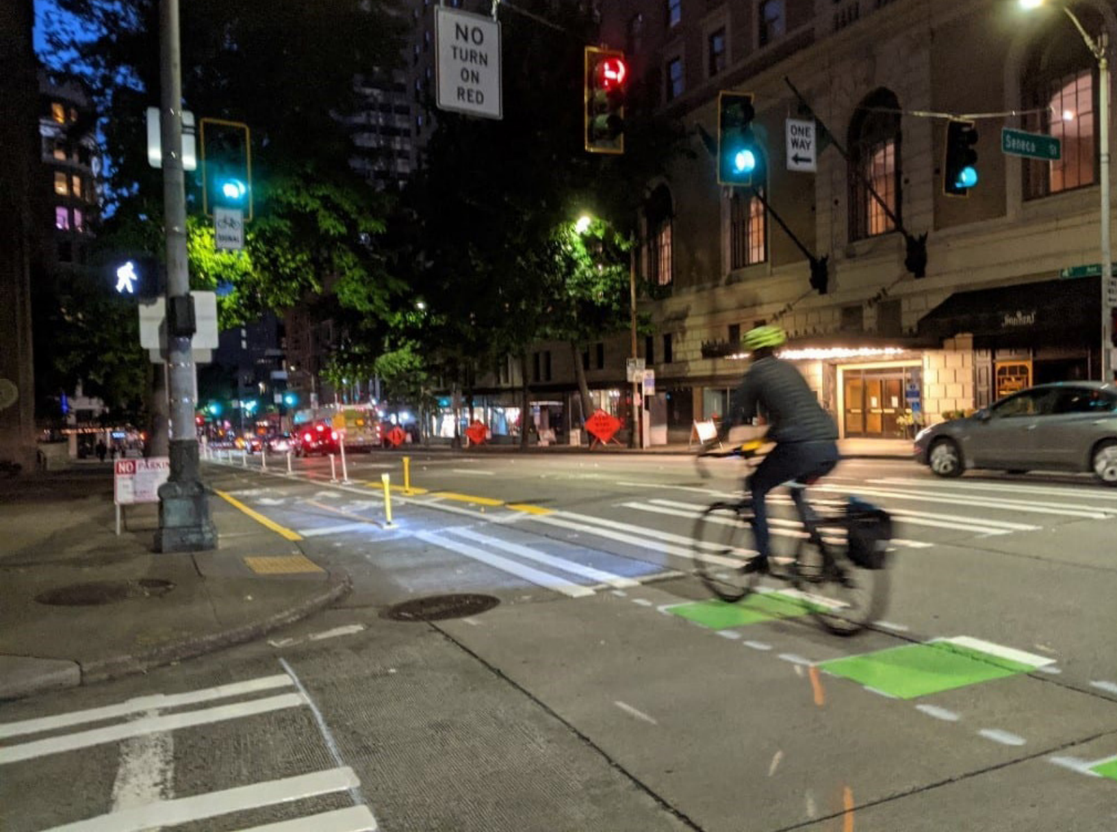
Fall 2020, 4th Ave protected bike lane
