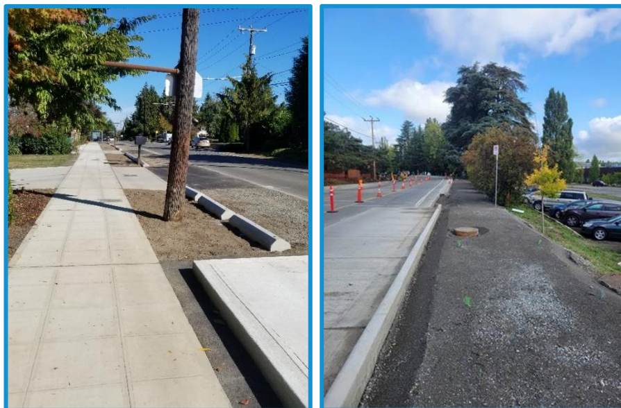
Program 25 | New walkway on 15th Ave NW (left); construction on sidewalks on Sand Point Way (right).
