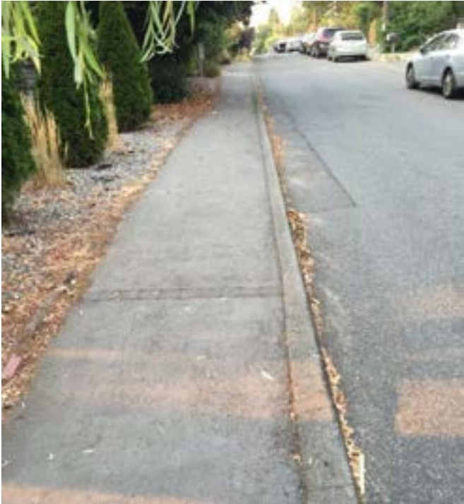
4.b. Stained asphalt sidewalk with curb (raised walkway)
