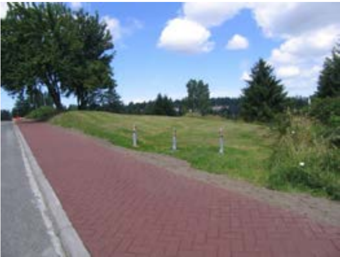
4.a. Stamped and stained asphalt sidewalk with curb (raised walkway)
