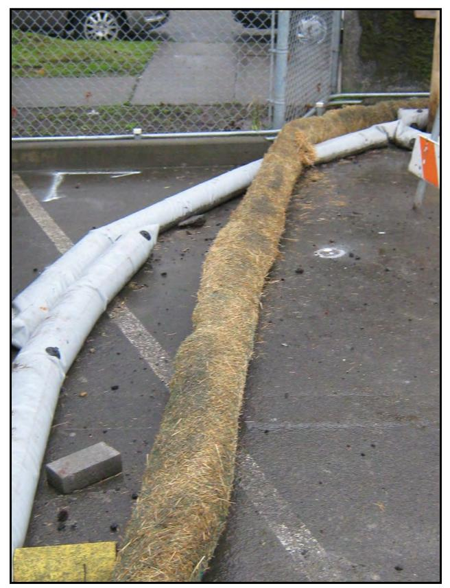
Figure 16. Curb and Gutter Barrier.
