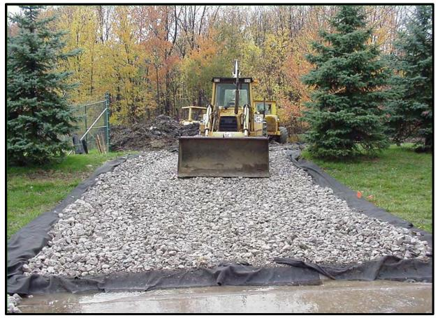
Figure 6. Stabilized Construction Access.
