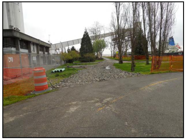
Figure 7. Stabilized Construction Access.
