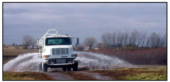
Figure 11. Using a Water Truck for Dust Control.
