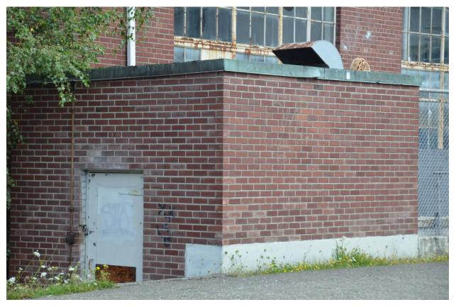
Building 119 was built between 1939 and 1944 and housed aircraft dope, a plasticized lacquer that was applied to aircraft fabric. Located near the assembly and repair building for easy access, it was separate due to the flammable nature of the dope.
