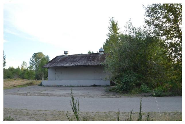
Building 312 is a concrete building with a loading dock that was constructed to hold small arms. Similar to other magazines, it was constructed far from daily operations and core functions of the base, and had road access for easy loading and unloading. However, due to the smaller nature of explosives that were housed here, it is an above-ground storage, as opposed to underground storage such as buildings 19, 54, and 55.
