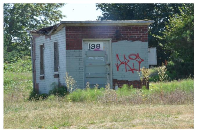
Building 98 was built somewhere between 1939 and 1943. It housed gas pumps that served the tank farm on the hill nearby, pumping fuel to the gas station on the base. This small building is divided into two rooms, each housing a pump.
